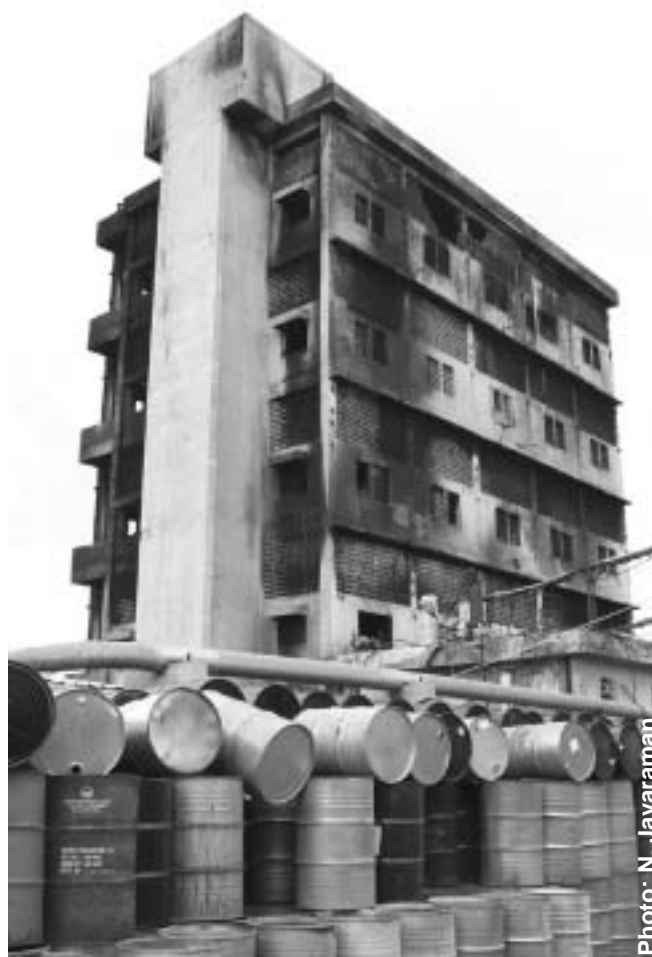
The Burnt Endosulfan Plant
